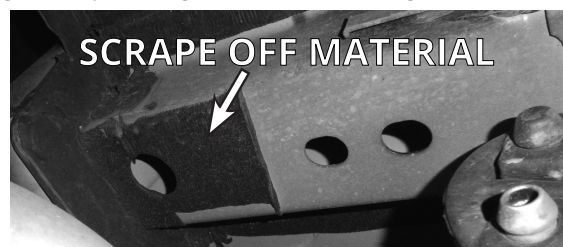
FIGURE A2: VIEW UNDER CHASSIS CHANNEL
