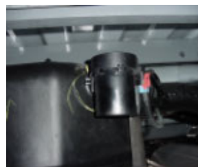
Figure C1, Step 1: Locate the Fuel Valve.
